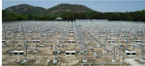
Figure 2. The antenna array and the TR modules, each feeding one antenna, of the MST radar.
