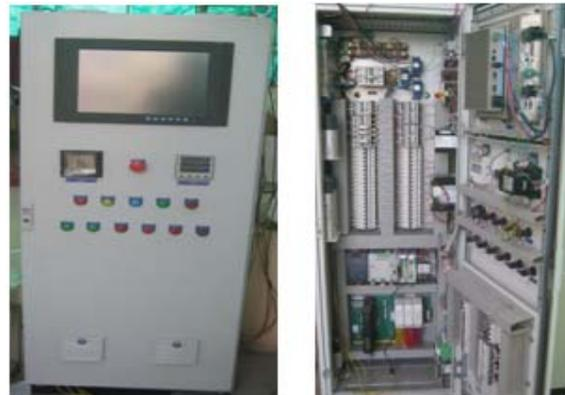
Figure 3: PDP Rack in Arudhra
